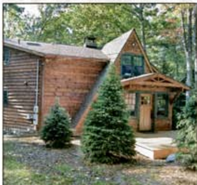
Clemleddy Construction's expertise and green building principles changed a simple seasonal A-frame into a custom year-round residence.
